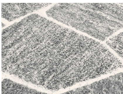
Bodenplatten formwild (polygonal)
